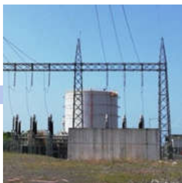
Substation Portico
