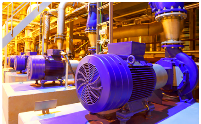
Figure 1: Electric motor as possible cause
